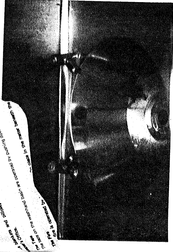
6.6 Contrasting Designs for "Push" Faucets. The faucets A (above) in the Rammoor dormitory at the University of Sheffield give little clue to their mode of operation. As a result, occupants must be supplied with the instruction sheet for "the taps". The faucets B (below) on the sink of a commercial airline are designed properly. Pushing is clearly indicated. No instruction manual is required.
