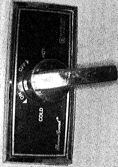
6.8 Simpler Faucets. In A (above) the mapping problem is solved—the faucet is presumed to be easy to use. The problem is that you cannot control the amount of water. On top of that, once the knob has been turned 180°, it is no longer clear which way to turn it in order to make the water hotter or colder. Faucet B (below) couldn't be simpler. It certainly is easy to use. Of course, you can only turn it on; you get a fixed temperature and a fixed volume of water.
