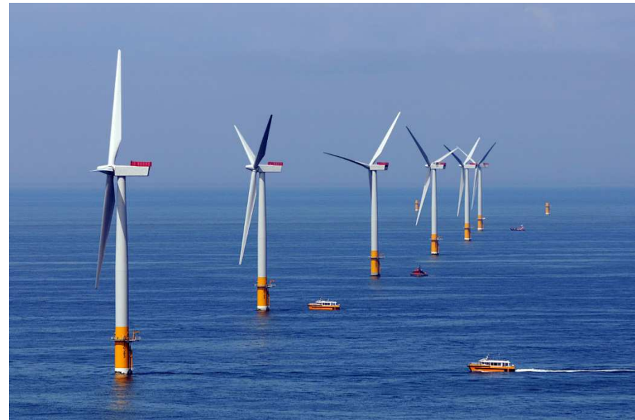
“Offshore” Greater Gabbard, UK 504 MW
